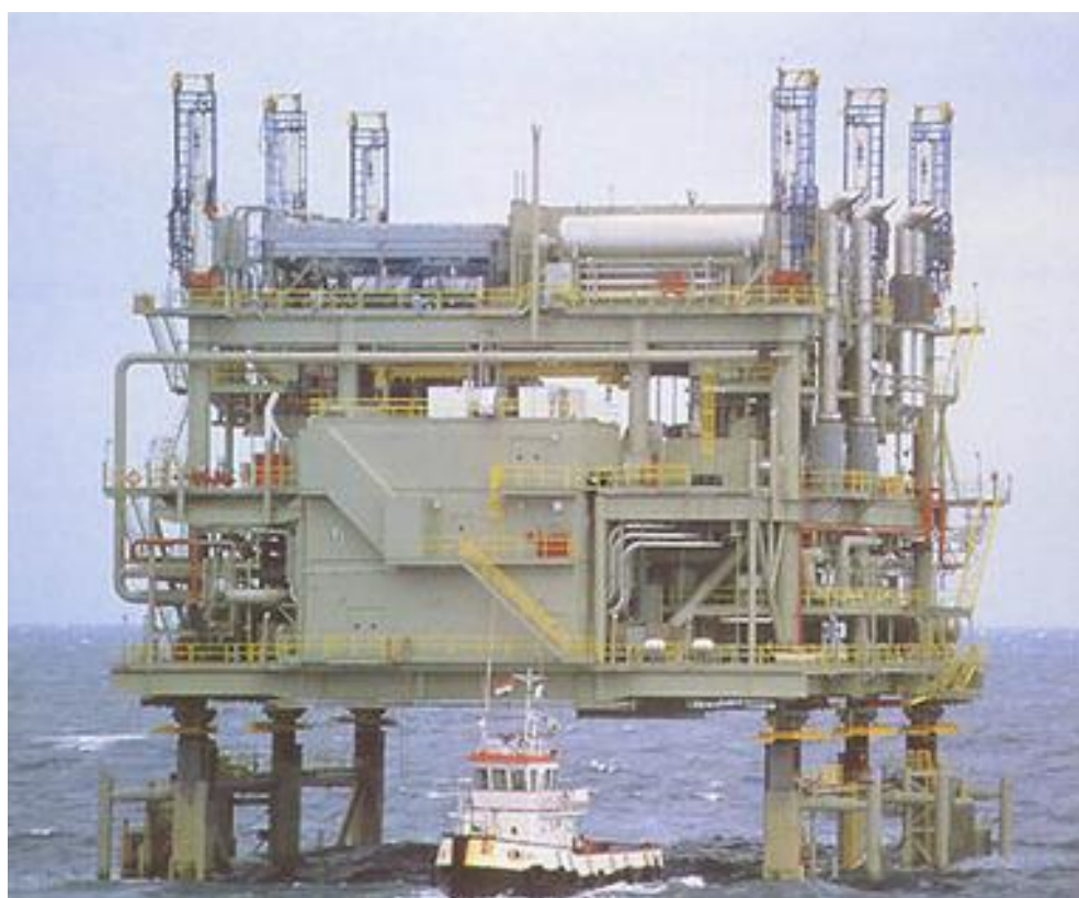
Image from http://www.offshore-technology.com/projects/ekpe/images/ekpe5.jpg (Accessed 2008)
