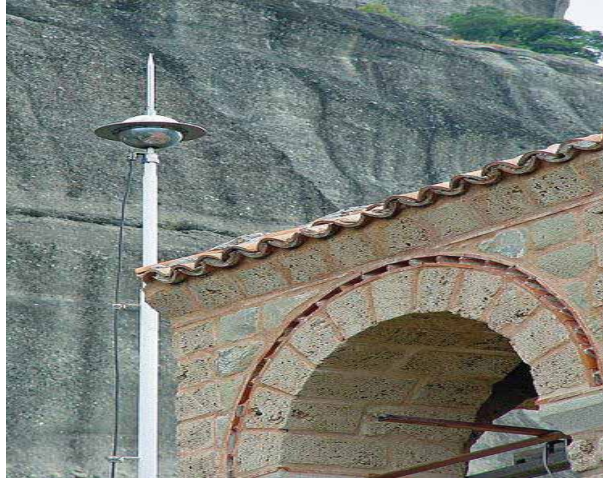
Figure 8: Lightning conductor at a church accessed from Wikimedia Creative Commons, 2010.
